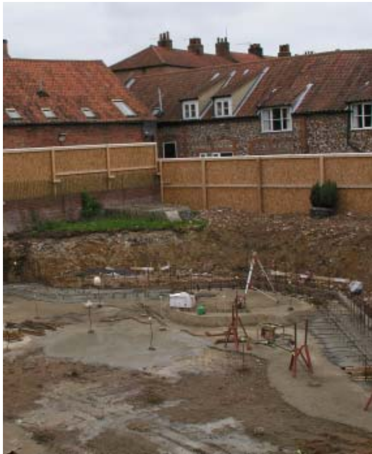
Work in progress - the sanctuary of the new church
